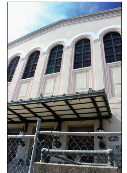
3: View of former Arena entrance (east facade).
