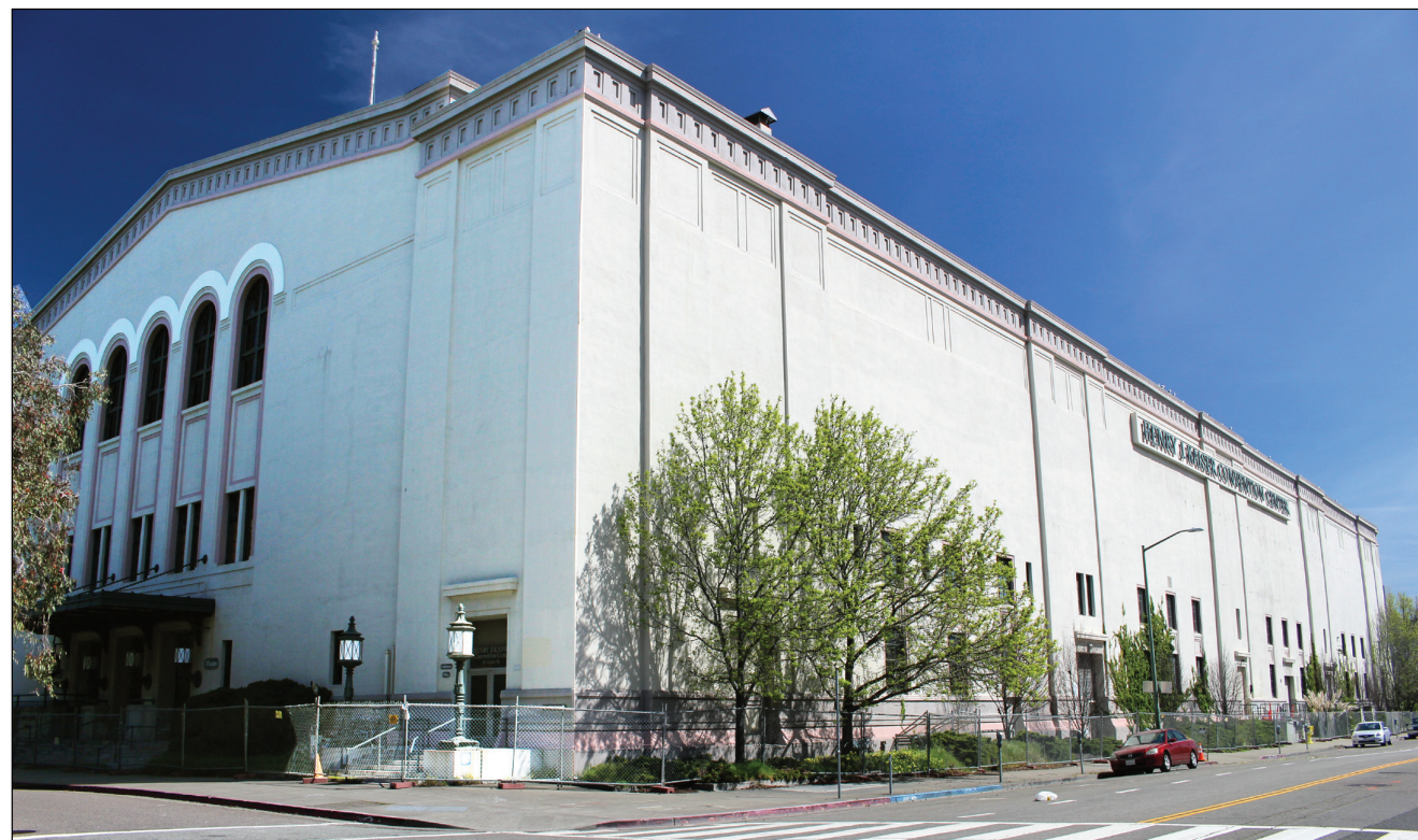
6: View of building rear (south facade) and Calvin Simmons Theatre entrance (west facade) from 10th Street.
