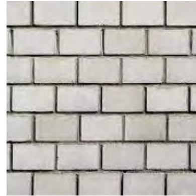
CONC. PRE-CAST W/ INTEGRATED COLOR & TEXTURE
