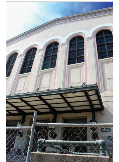
3: View of former Arena entrance (east facade).
