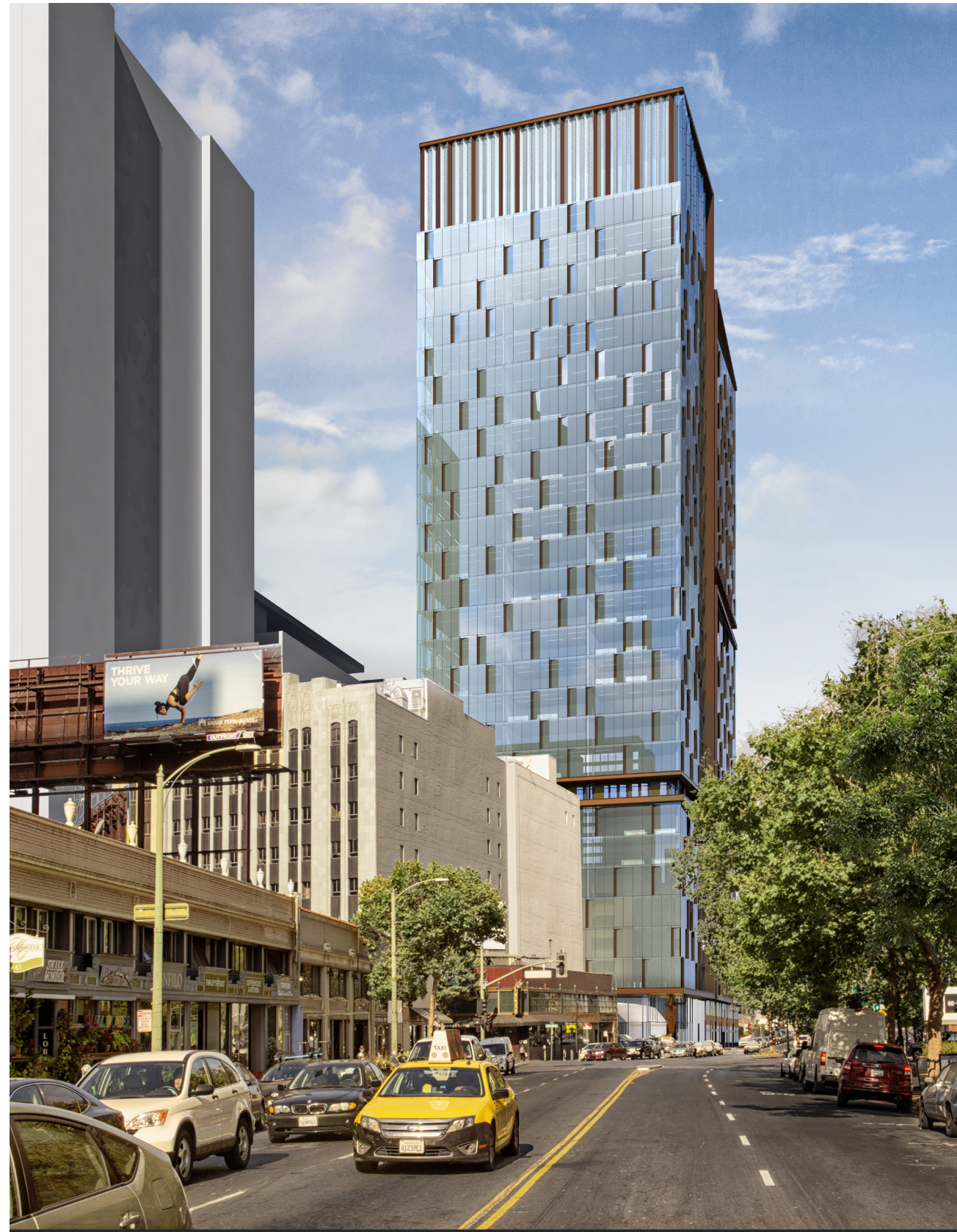
EAST ELEVATION FROM GRAND AVENUE AND BROADWAY
