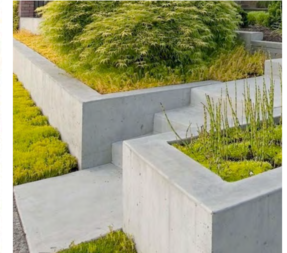
EXAMPLE - CAST IN PLACE PLANTER BOX
