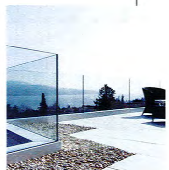
ROOF DECK GLASS RAILING
