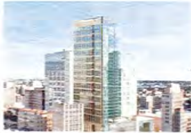
1640 BROADWAY Lennar 380' Under Construction
