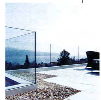
ROOF DECK GLASS RAILING
