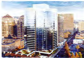
601 CITY CENTER Shorenstein 24 story Under Construction
