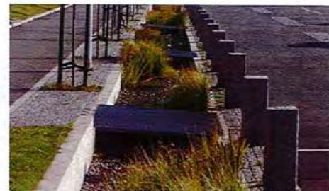
BIORETENTION BASIN w/ METAL GRATE
