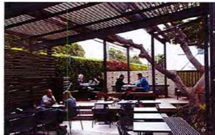
OVERHEAD PERGOLA STRUCTURE
