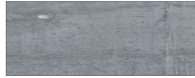
C1 CONCRETE - EXPOSED
