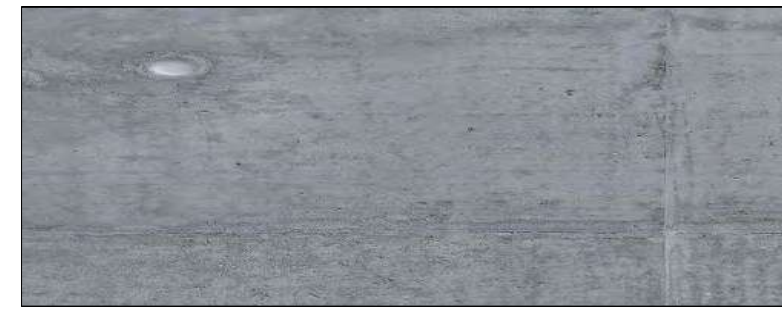
C1 CONCRETE - EXPOSED
