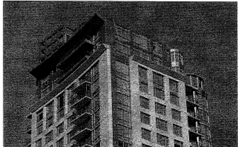
The topmost floors of towers should be architecturally differentiated through the use of setbacks, changes in material, building shape, etc.
