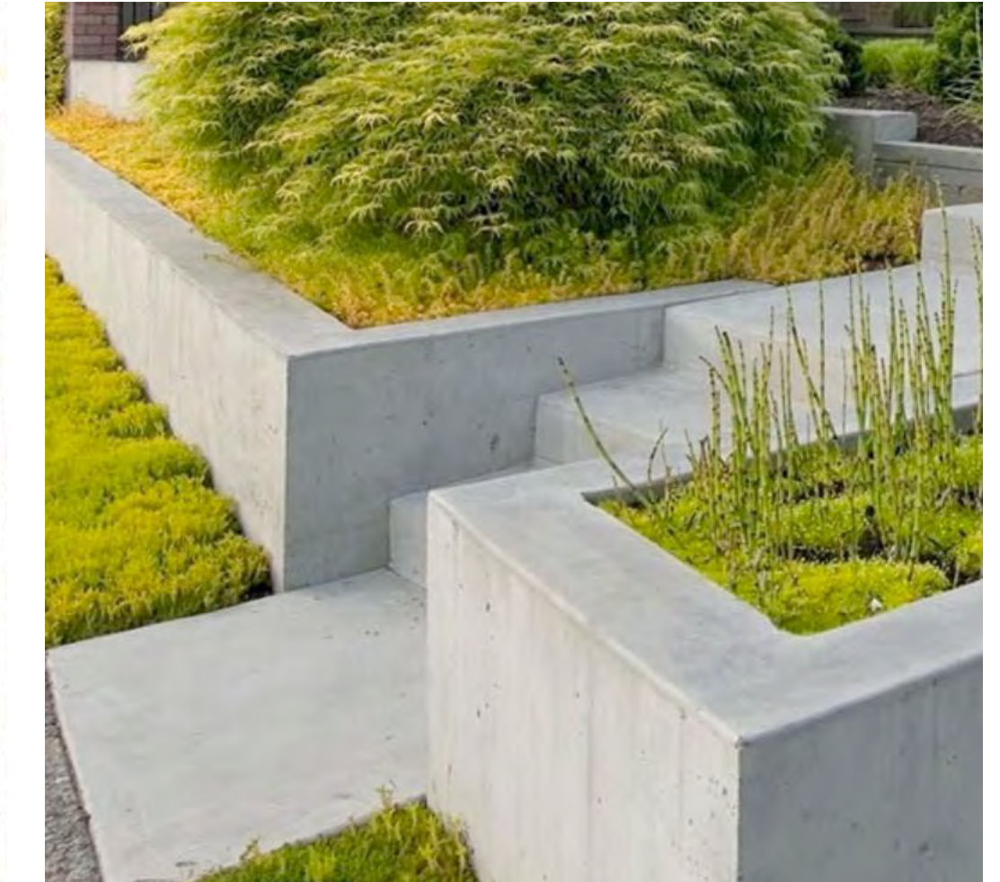
EXAMPLE - CAST IN PLACE PLANTER BOX
