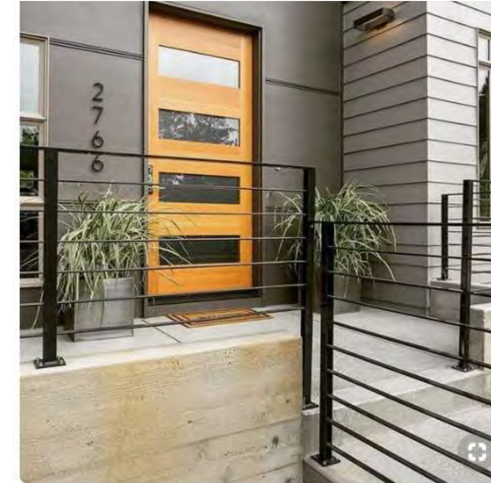
EXAMPLE - OPEN LINEAR RAILING @ CONCRETE STOOP
