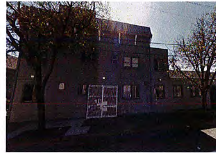
8 3267 & 3275 HOLLIS STREET, DOWN THE STREET FROM THE SITE
