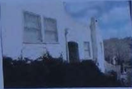
SIDE OF HOUSE - SOUTH ELEVATION
