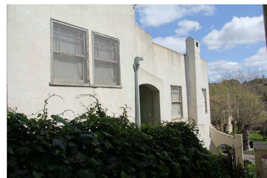
SIDE OF HOUSE - SOUTH ELEVATION
