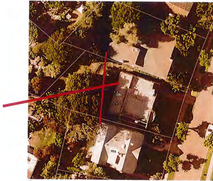
Figure 10 963 Grosvenor Place - Existing aerial site with adjacent parcels
