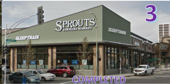
COMPLETED 3001 Broadway: 39,000 sf Retail
