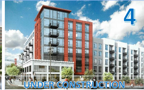
UNDER CONSTRUCTION 3000 Broadway: 127 Residential Units, 8,000 sf Retail
