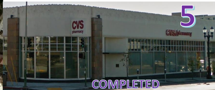
COMPLETED 2964 Broadway: 26,312 sf Retail
