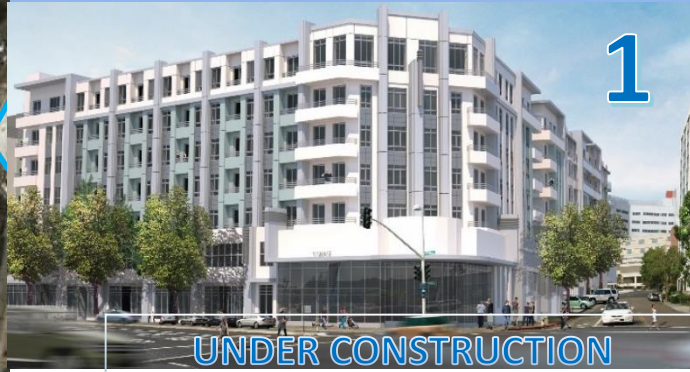
UNDER CONSTRUCTION 3072 Broadway: 432 Residential Units, 22,000 sf Retail
