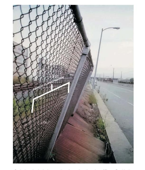
Geologic and seismic damage along the northern boundary of Burma Road in the Gateway development area. To the left is a fence and sidewalk, demonstrating that substantial settlement has occurred in the area. The top of the East Bay Municipal Utility District outfall pipeline is to the left of the fence. This pile-supported structure has remained stable, while surrounding fill has not.
