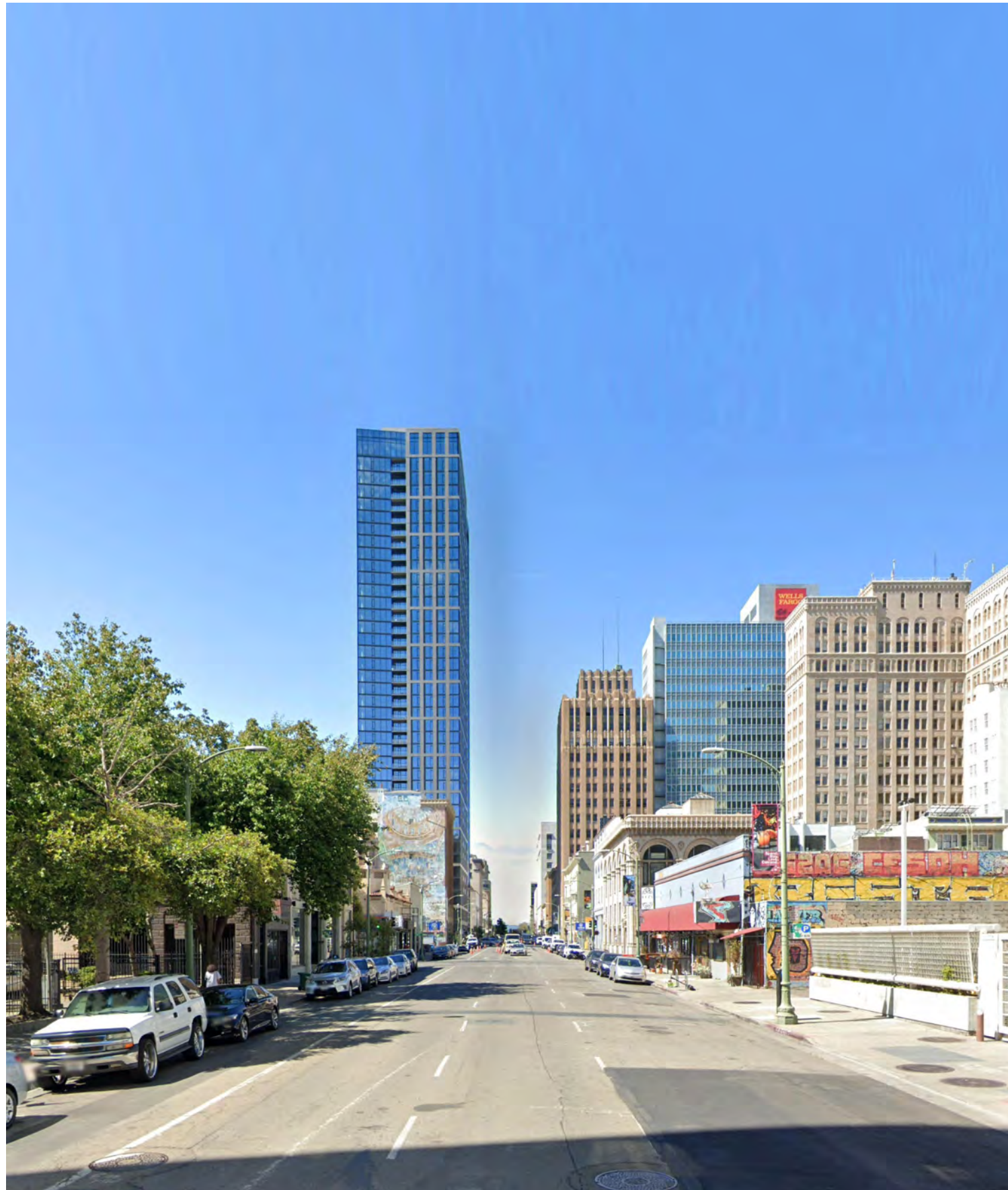
VIEW FROM CITY FRANKLIN LOOKING SOUTH
