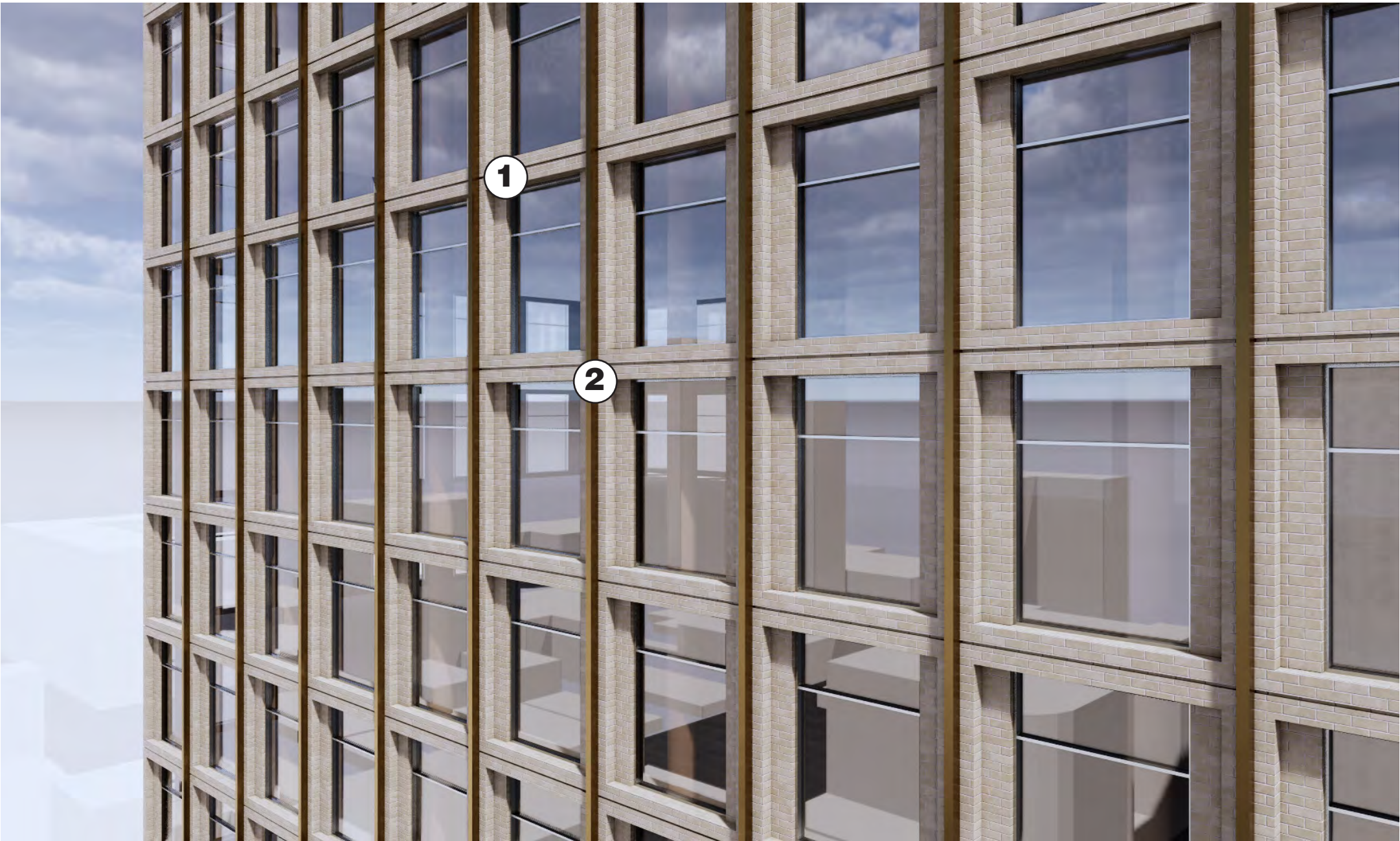
1. BEIGE BRICK VENEER ON PRECAST PANEL 2. BRONZE METAL FINIS
