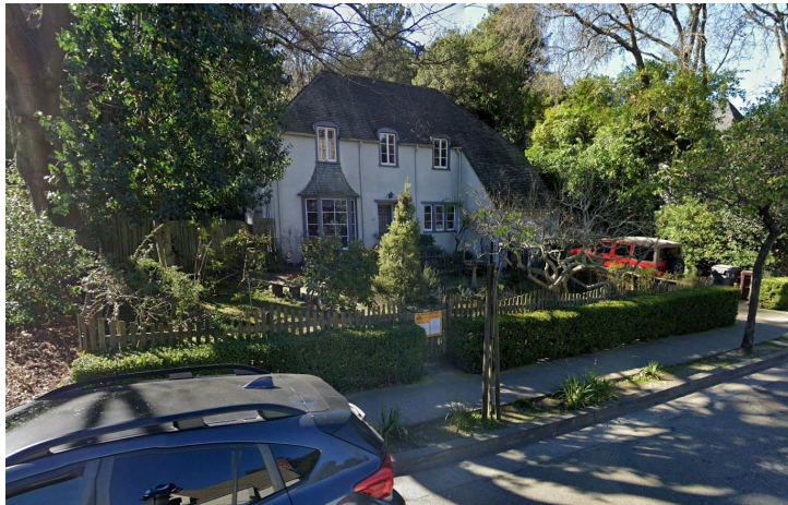
View looking northwest at 901 Trestle Glen
