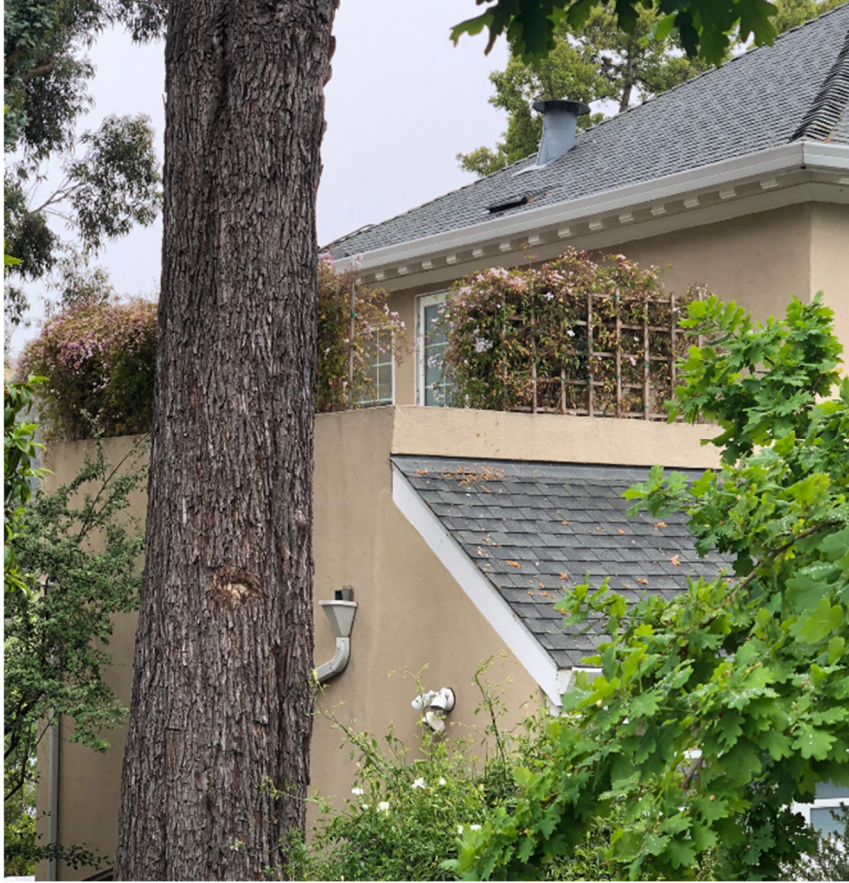
Figure 7a: 671 Longridge Road, Northeast Façade, 2021
