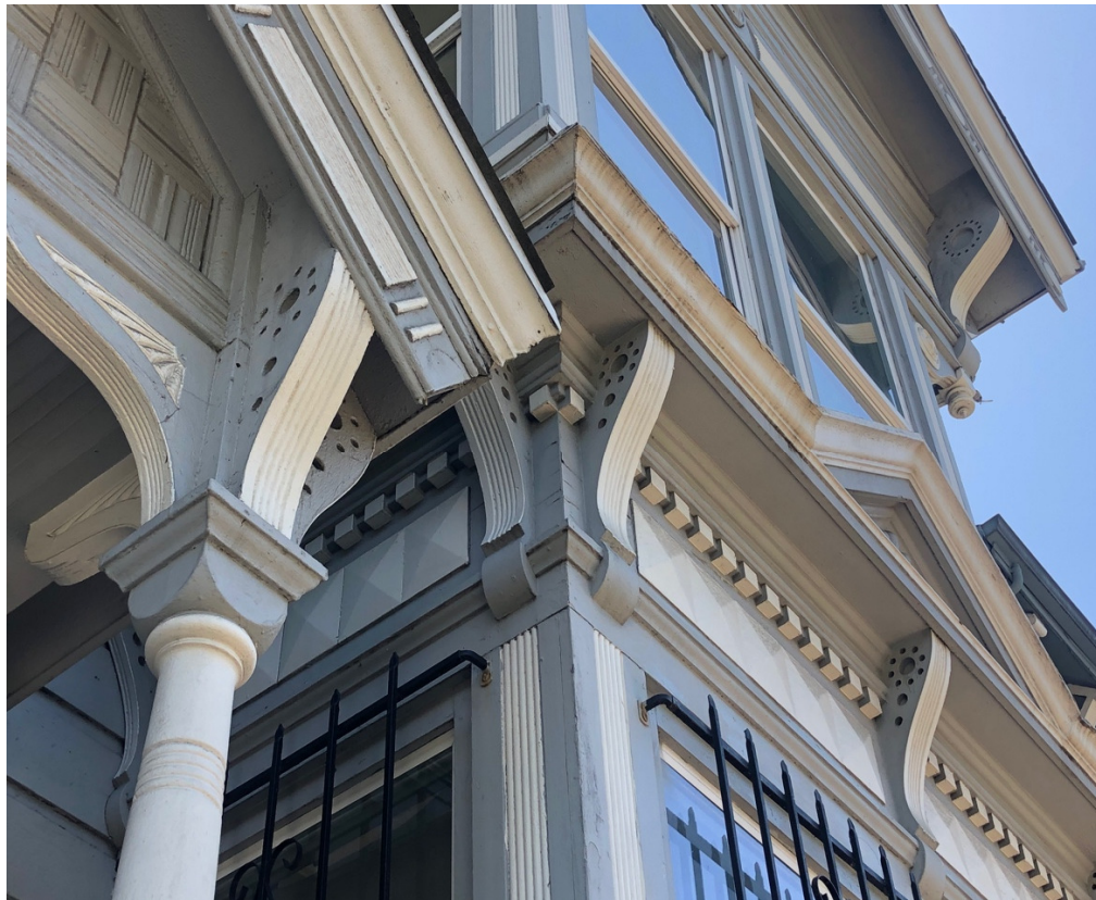
Geometric perforated brackets, small under 1 st story eaves, large under the roof line; checkerboard and wing motifs in porch gable (at left)
