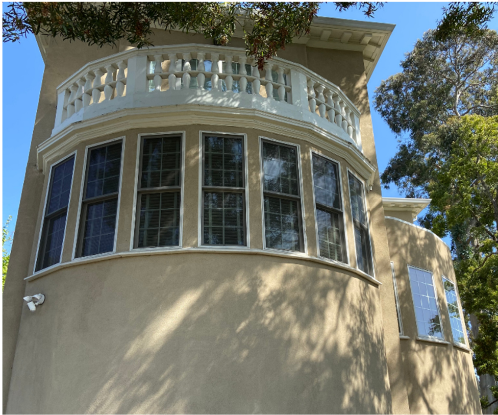
Figure 5a: 671 Longridge Road, West Façade, 2021
