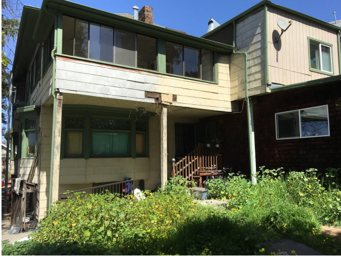
back of house facing east, exterior porch on upstairs unit
