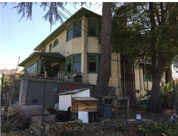
southwest corner of house
