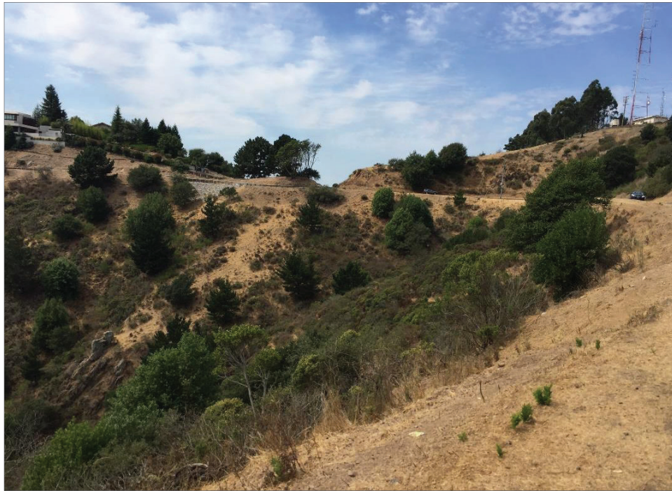
Existing Condition. Area along Grizzly Peak Boulevard looking west.
