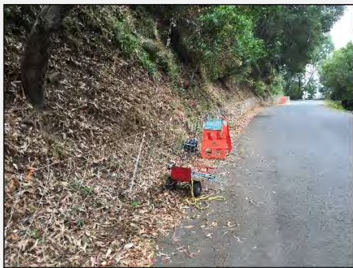
Exhibit 2. Fencing installed along roadway for grazing management.
