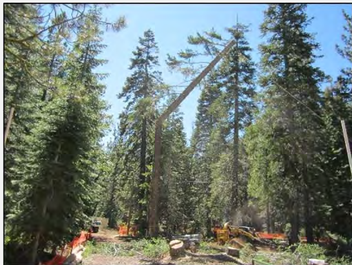
Exhibit 10. Tree being removed in segments.
