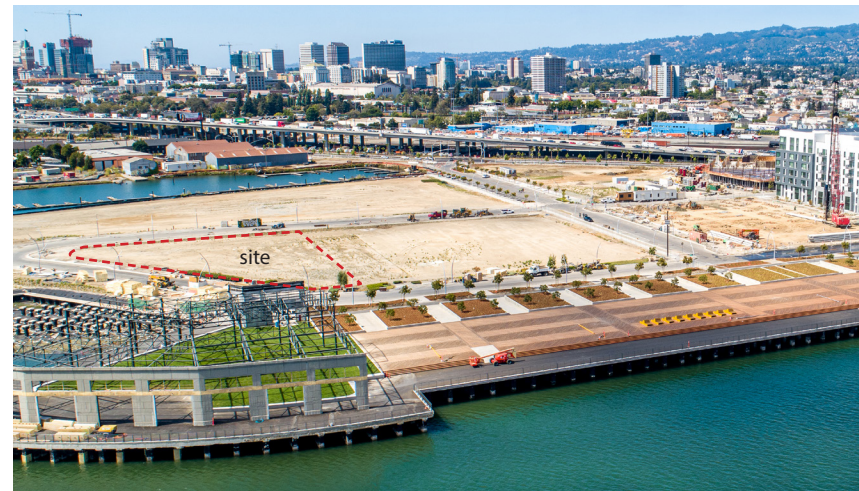
A. Aerial View Looking North
