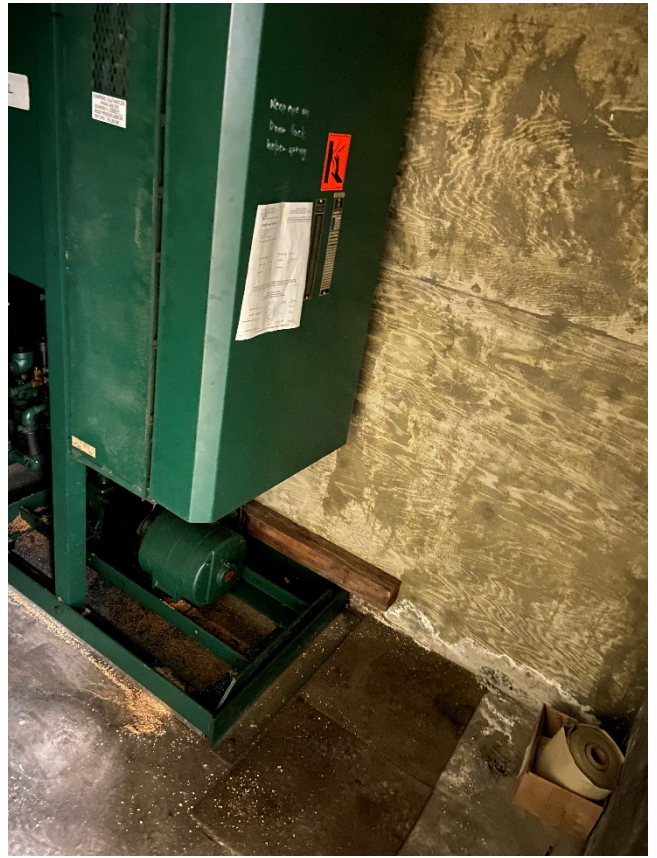
Photograph 9: Mechanical room in the basement with odors as well as staining and absorbent on the floor.
