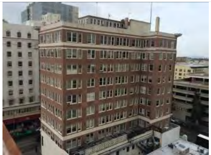
48. Additional building to the west - facing southwest
