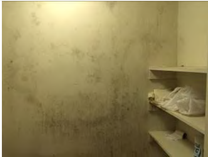
33. Microbial growth in the 5 th floor janitorial closet
