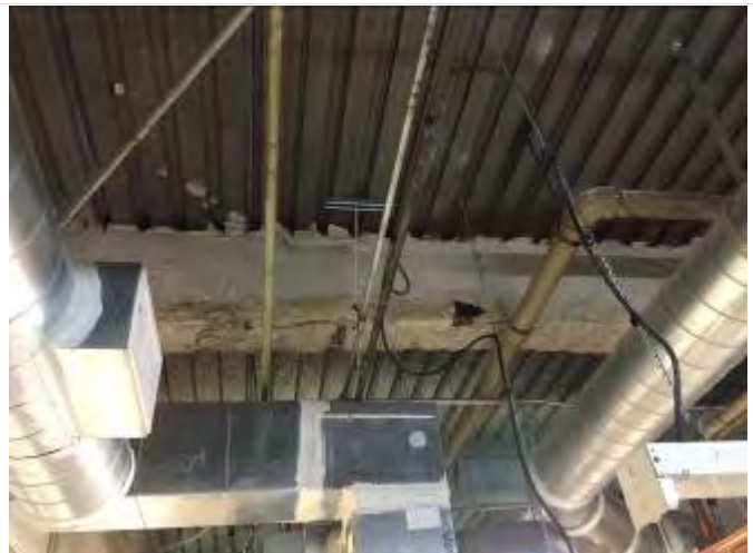
24. Ceiling area of Room B05 (spray-on fireproofing on beams visible)
