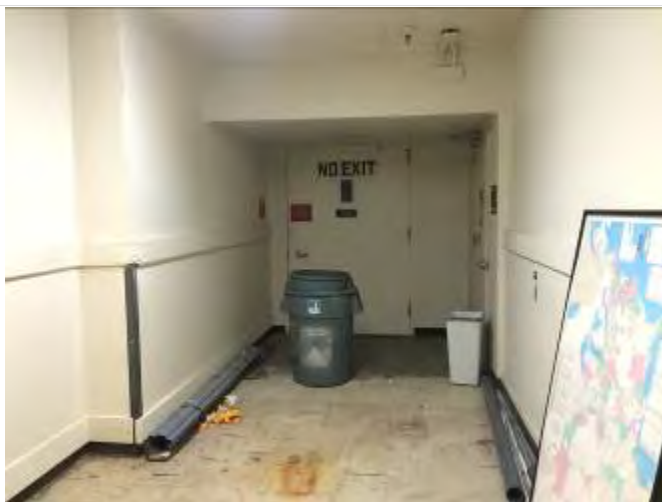
17. Basement emergency exit area with older floor tile
