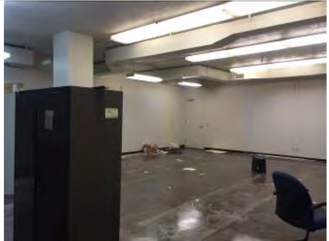
20. Basement Storage Room – B17
