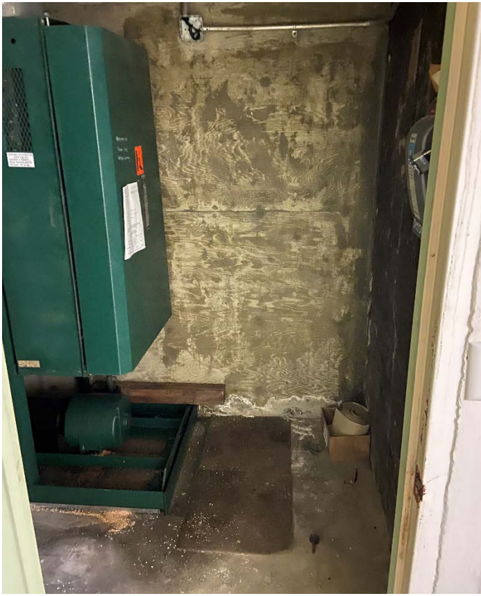
Photograph 9: Mechanical room in the basement with odors as well as staining and absorbent on the floor.
