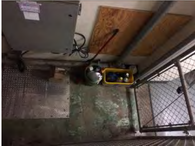
13. Cleaning supplies under stairwell to basement area
