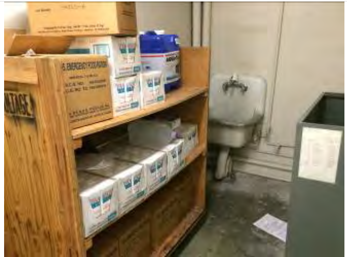
22. Basement Janitorial Room – B06
