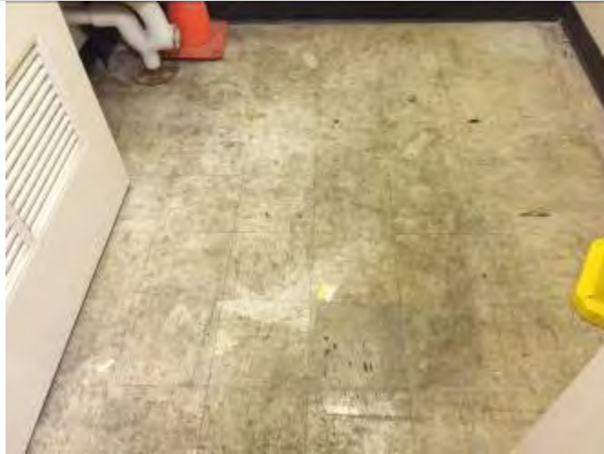
31. Typical flooring in janitorial closet (4 th floor)
