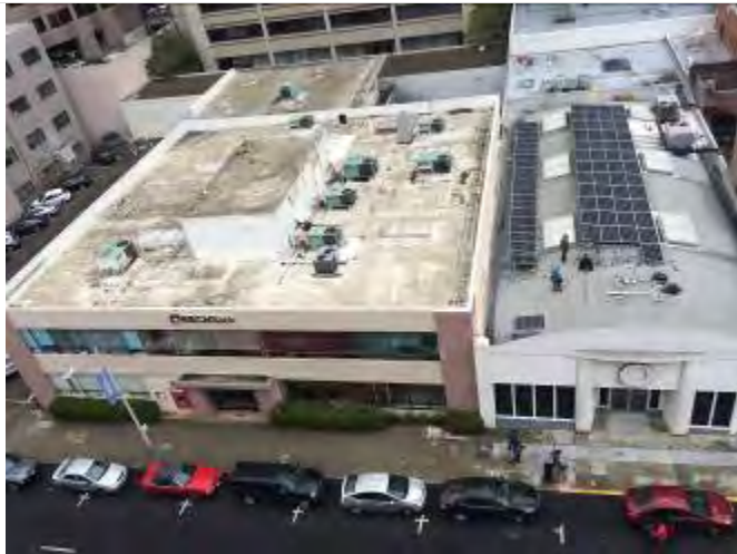
45. Adjacent buildings to the east, across Webster Street – facing east
