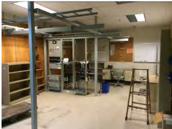
35. Second floor former telecom room
