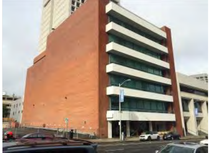
2. East and south sides of building – facing northwest
