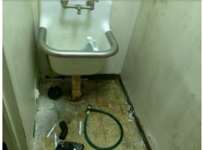
32. Fifth floor janitorial room
