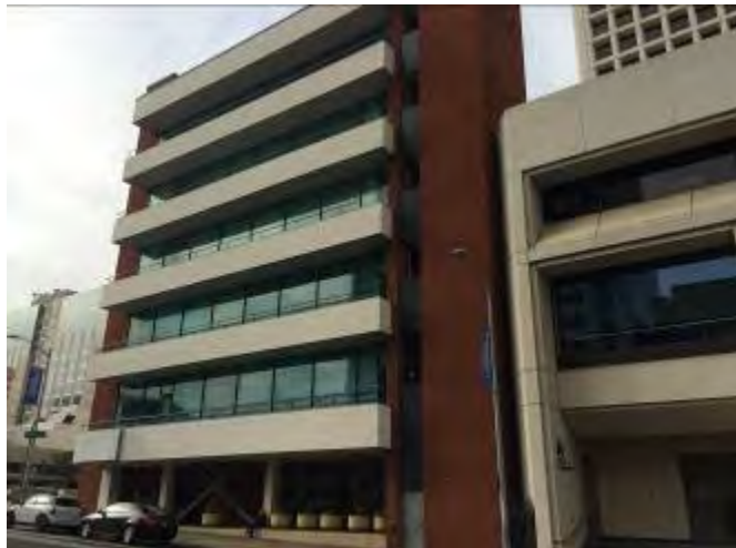
1. Front of building – facing west
