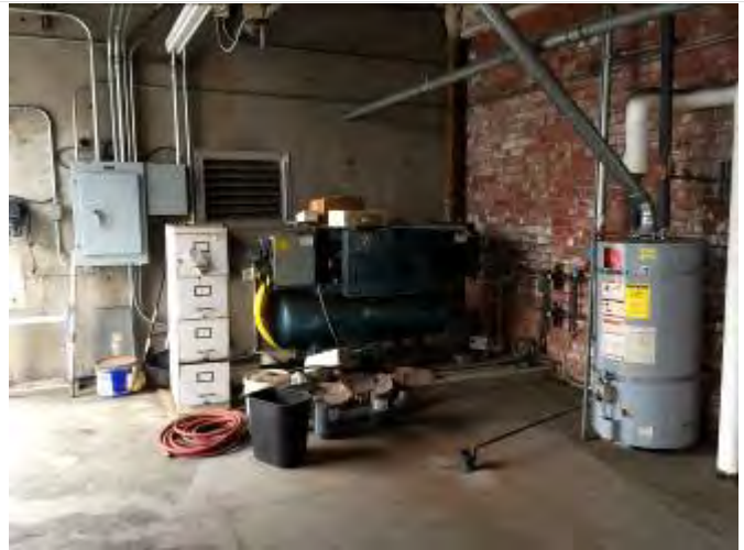
38. Water heater and other rooftop electrical equipment
