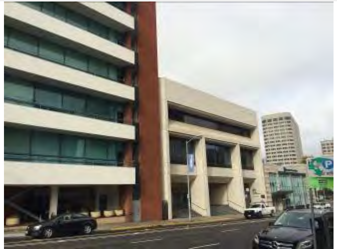
44. View of adjacent building to the north – facing northwest
