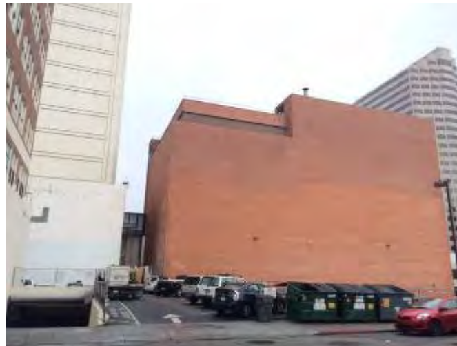
3. South and west sides of building – facing north
