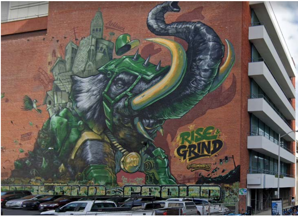
Photograph 1: Six-story vacant building at 1919 Webster Street.
