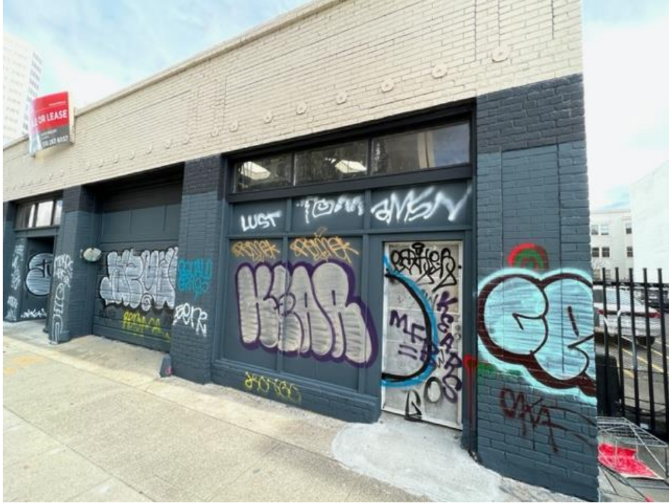
Photograph 5: Close-up of the front façade of 1600 Harrison Street looking east.
