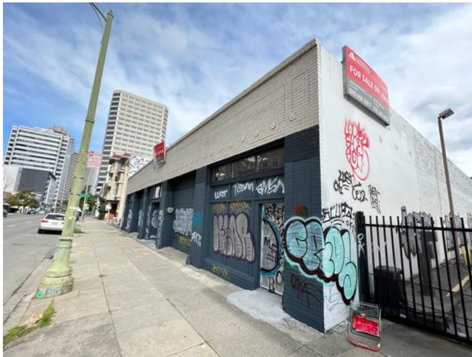
Photograph 4: View looking north at the front façade of 1600 Harrison Street.
