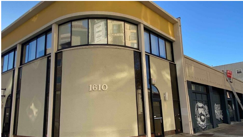
Photograph 1. Northeastern adjacent commercial offices
