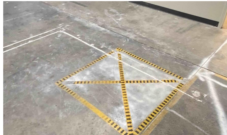
Photograph 10. Unknown floor marking located in southeastern corner of commercial office space
