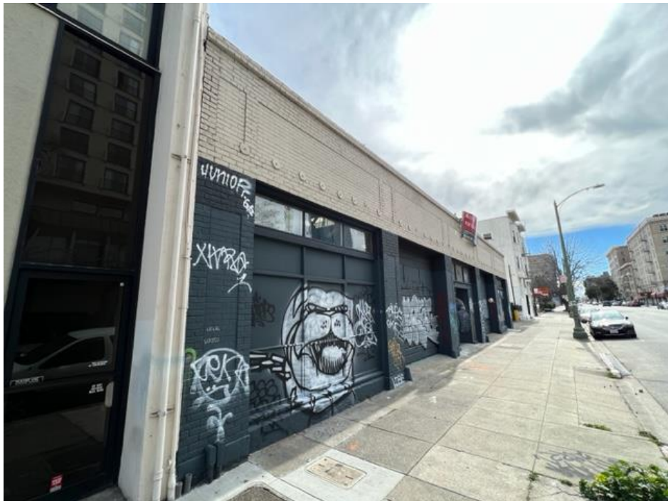
Photograph 6: Close-up of the front façade of 1600 Harrison Street looking south.
