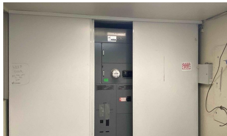
Photograph 12. Utility hookups on subject property
