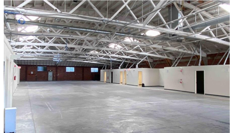
Photograph 6. Interior vacant office space
