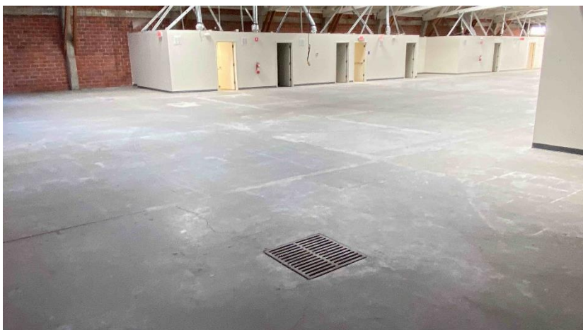
Photograph 11. Floor drain in the central area of the commercial office space
