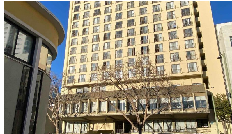
Photograph 2. Northwestern adjacent multi-family residences
