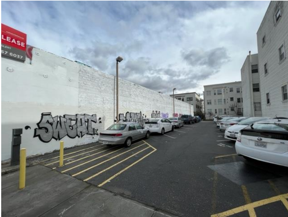
Photograph 3: View looking east at the south elevation of 1600 Harrison Street.
