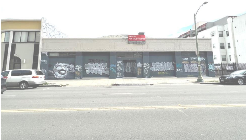
Figure 4: Photograph of 1600 Harrison Street in February 2023 illustrating front façade alterations.
