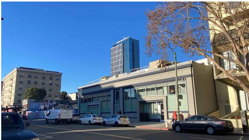
Photograph 3. Northwestern adjacent commercial offices
