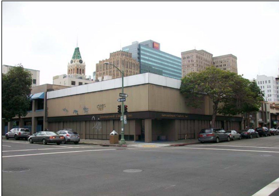
351-359 15 th Street, north and east façades. View to the southwest. 3/3/16.
