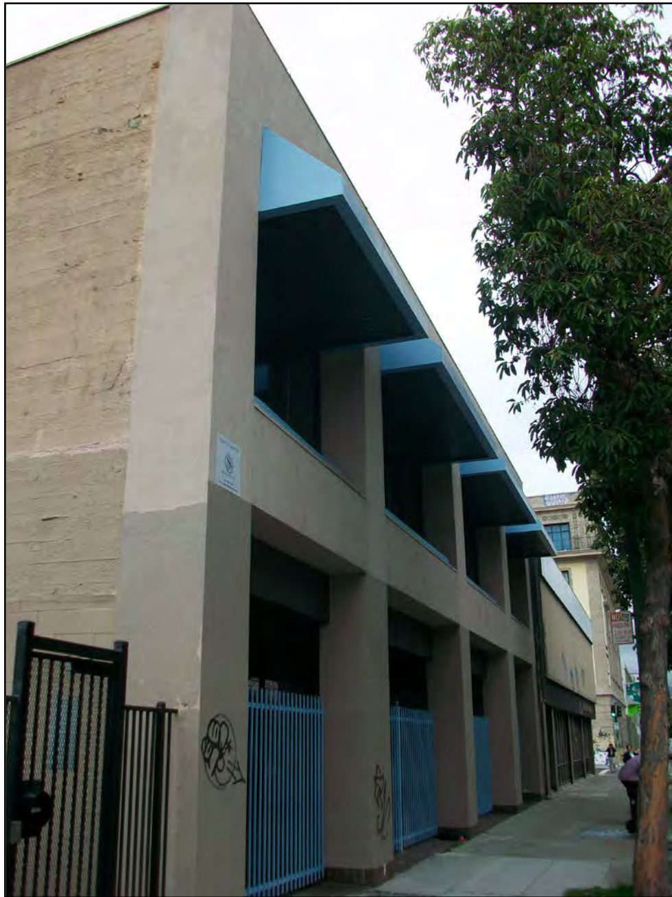
1433 Webster Street, east façade detail. View to the north. 3/3/16.
