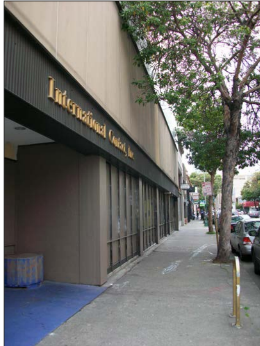
351-359 15 th Street, north façade detail. View to the west. 3/3/16.
