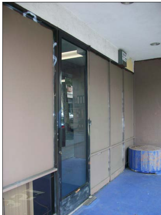
351-359 15 th Street, north façade detail. View to the southwest. 3/3/16.
