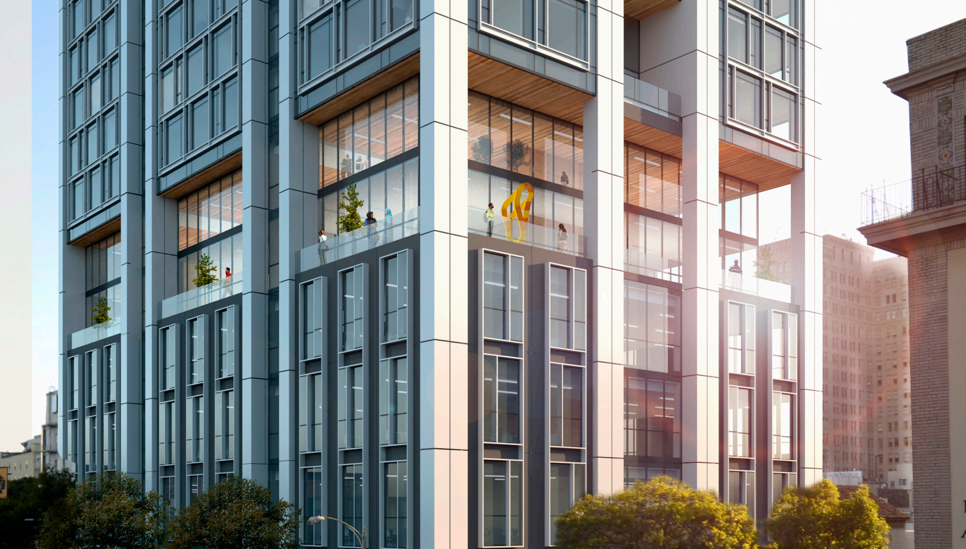
An expression of art is located in the deep recess on 15th street to pull the Oakland Art Walk up into the building.
