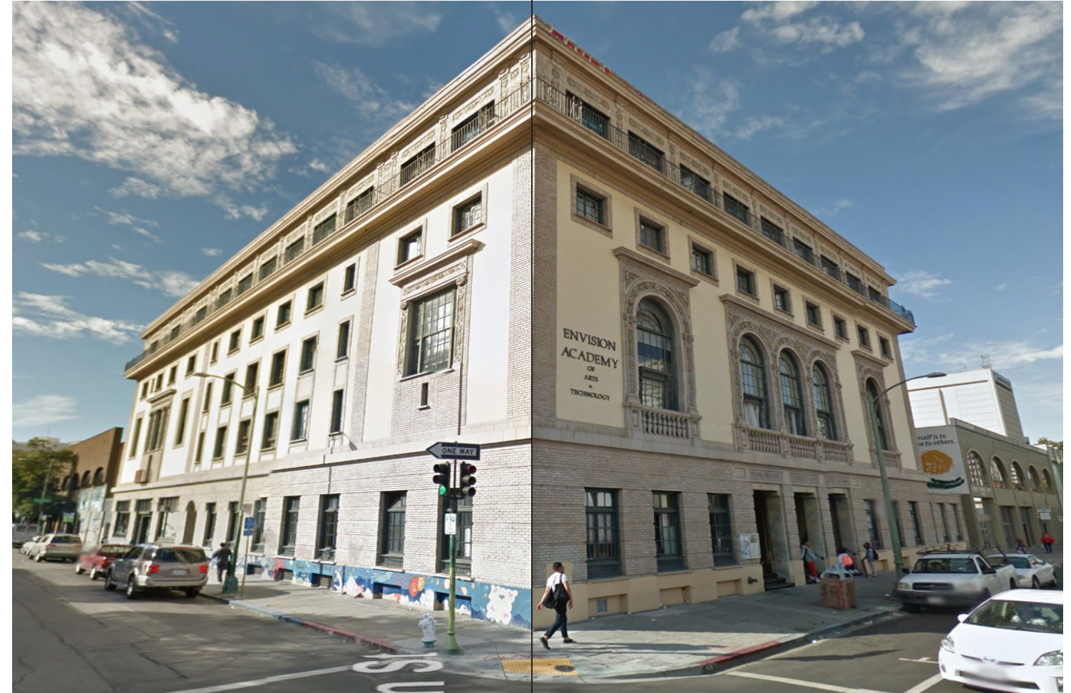
SIDE FACADE: South Facing
