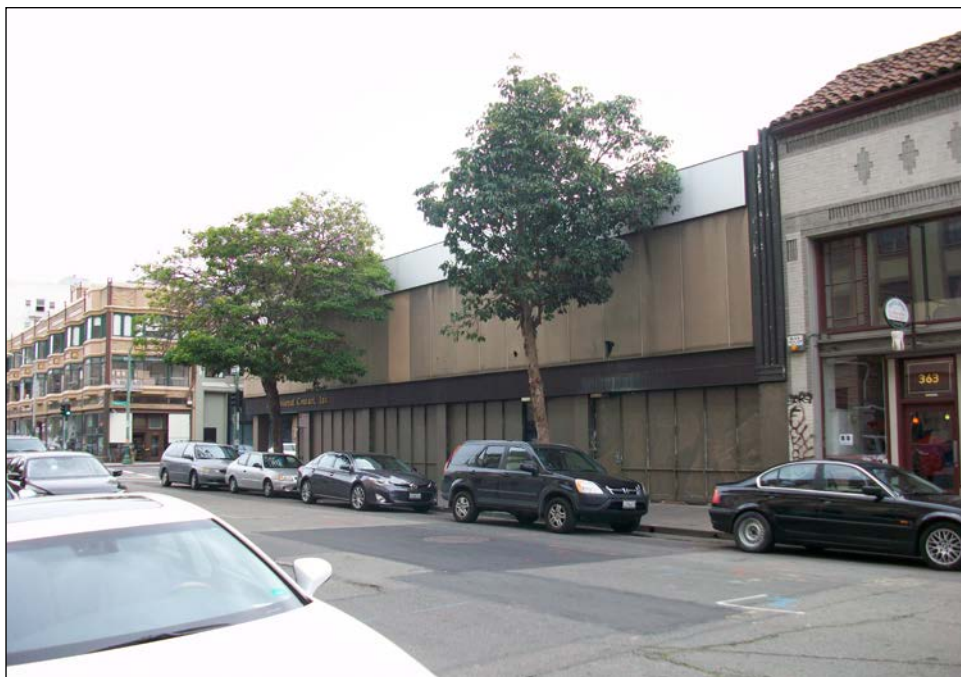
351-359 15 th Street, north façade. View to the southeast. 3/3/16.
