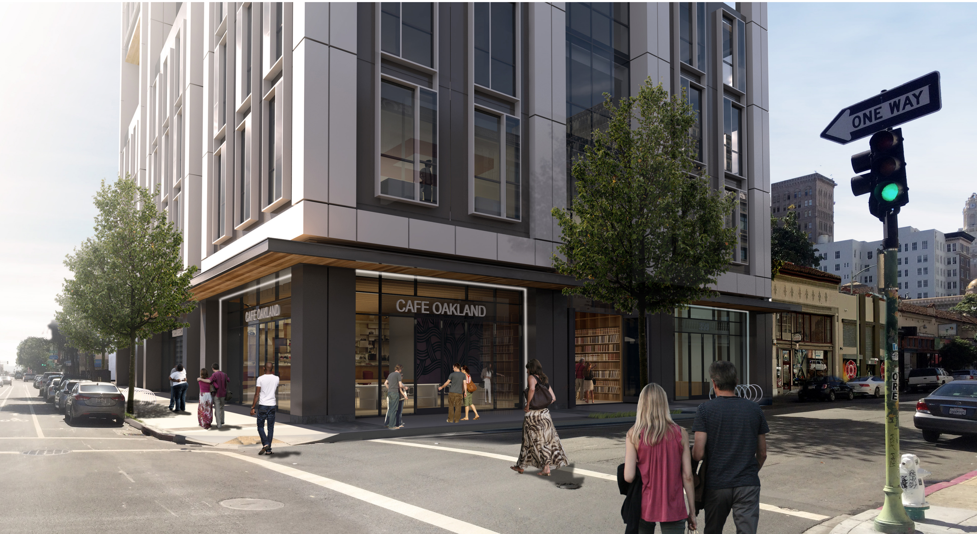
A wood clad canopy compresses the sidewalk along 15th street to establish a building base at the scale of the existing retail corridor
