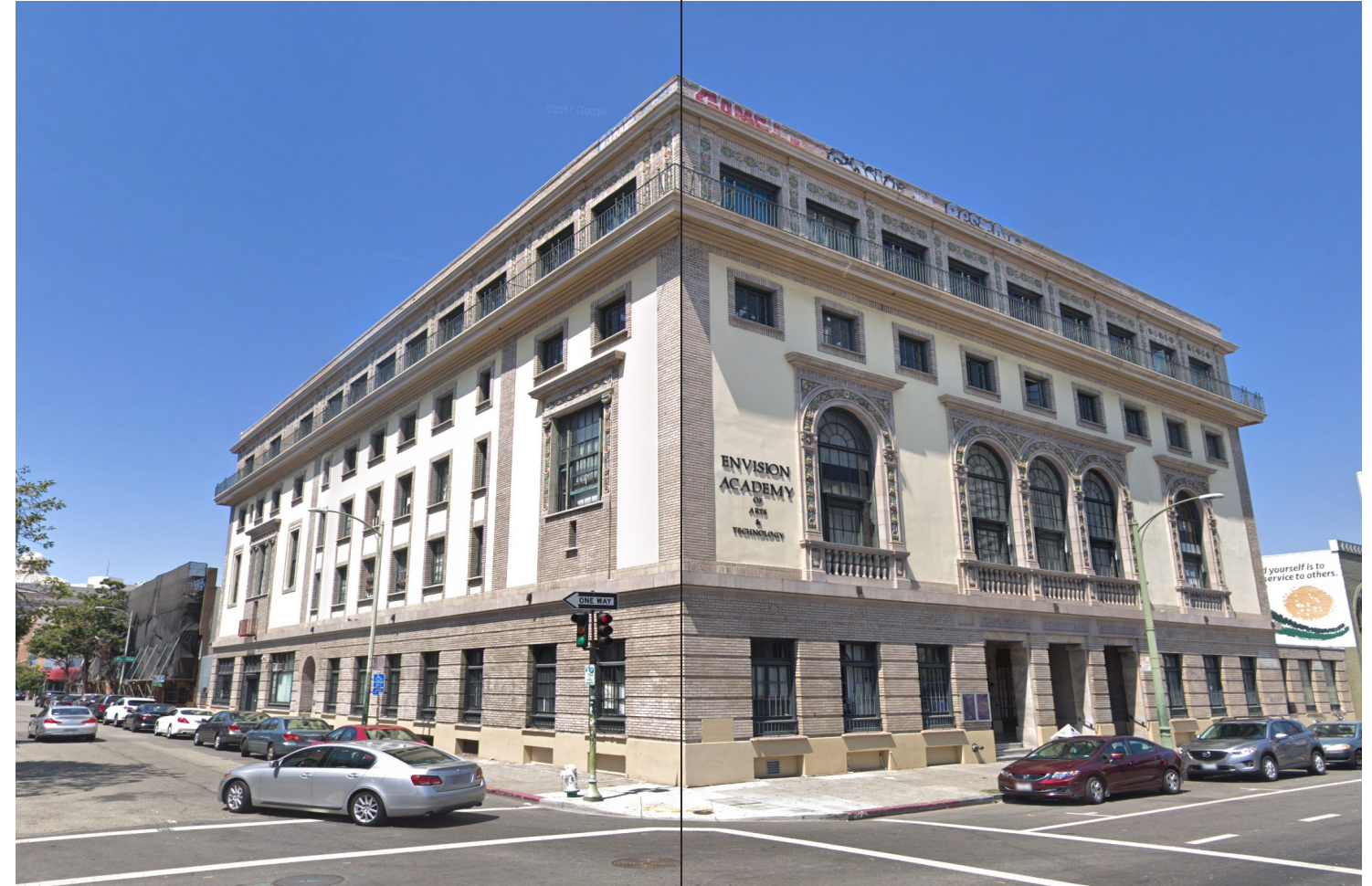
SIDE FACADE: South Facing
