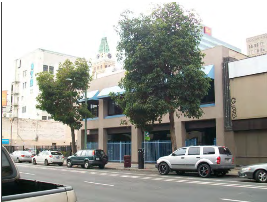
1433 Webster Street, east façade. View to the southwest. 3/3/16.
