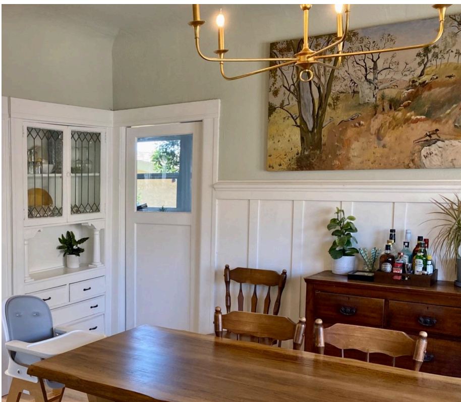
Dining room showing original built-in glass door hutch with miniature columns that was preserved during a kitchen remodel, and addition of salvaged door for doorway to laundry room, trim work, and beautiful original board and batten.
