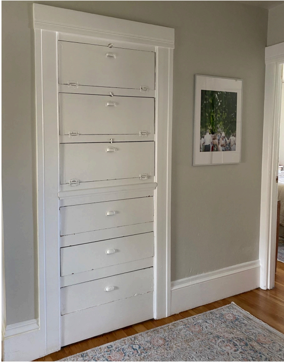
Upstairs built-in hallway storage showing original design and trims.
