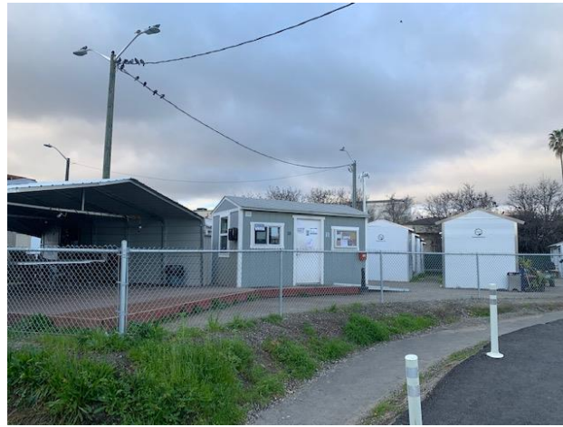
2. Cabin structures at the Site. View is from the east.
