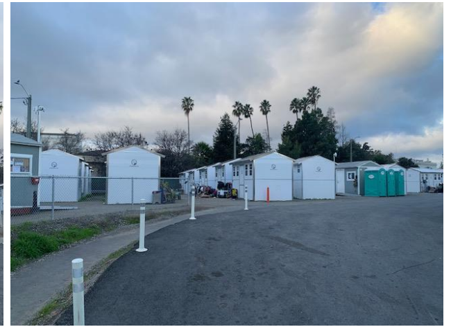
3. Cabin structures at the Site. View of from the east.
