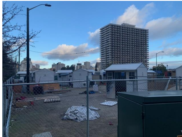
5. Cabin structures at the Site. View is from the south.
