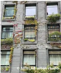
Figure 2.28: Examples of enhanced opening depth
