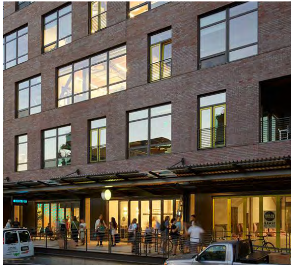
Work/Live units line the ground floor of this multifamily building
