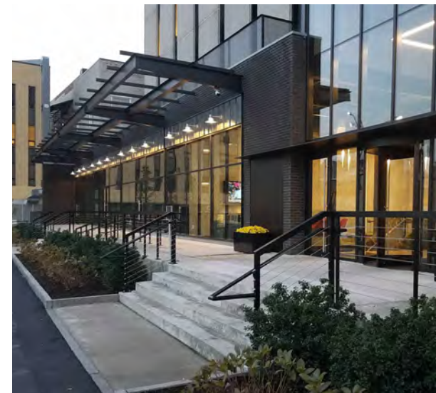
Central staircase and elevated walkway to enhance the commercial feeling of Work/Live units
