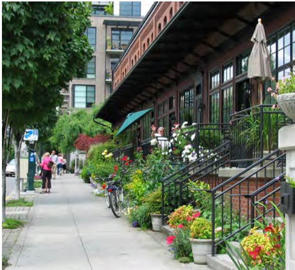
Ground floor work/live entries with terraces at 98th Avenue
