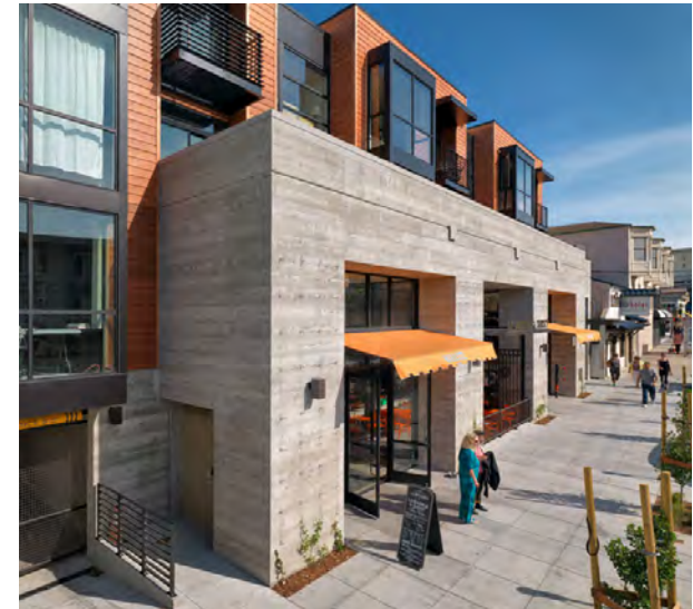
Commercial space entry
