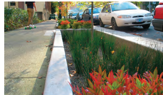
BIORETENTION PLANTING AT CURB
