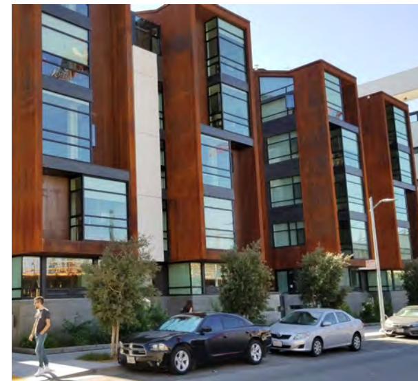
Building articulation through vertical bays and contrasting materials
