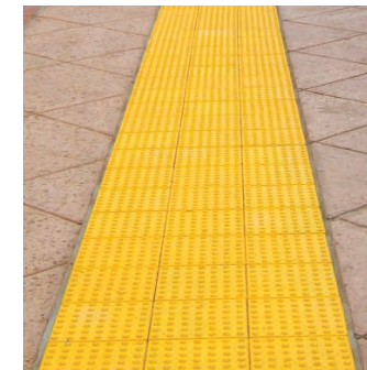
DETECTABLE WARNING TILES
