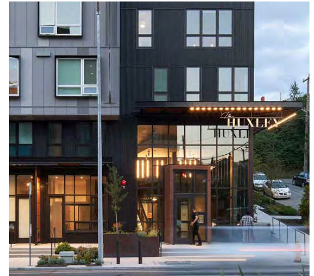
A corner entry invites residents into this apartment lobby entry
