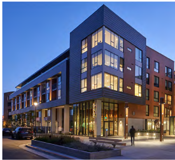
Main building entry corner
