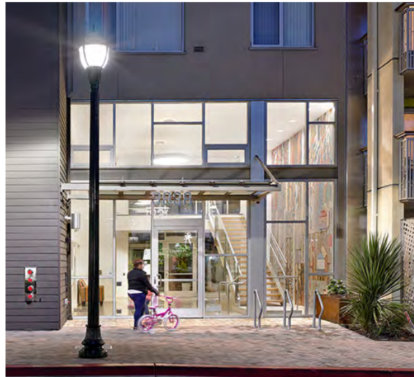
Multifamily building entry
