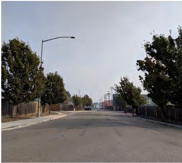
Blake Drive existing conditions
