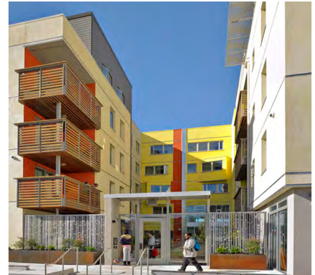
Metal and wood accents can provide texture and richness against stucco walls
