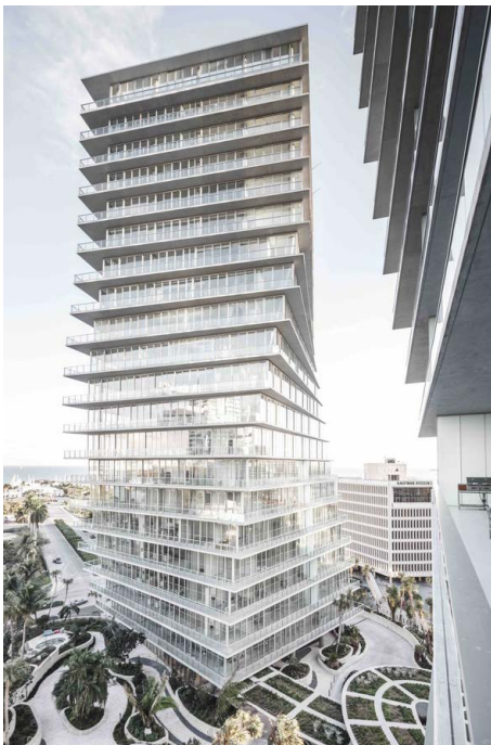
Figure 17: Shaping West Tower Facade
