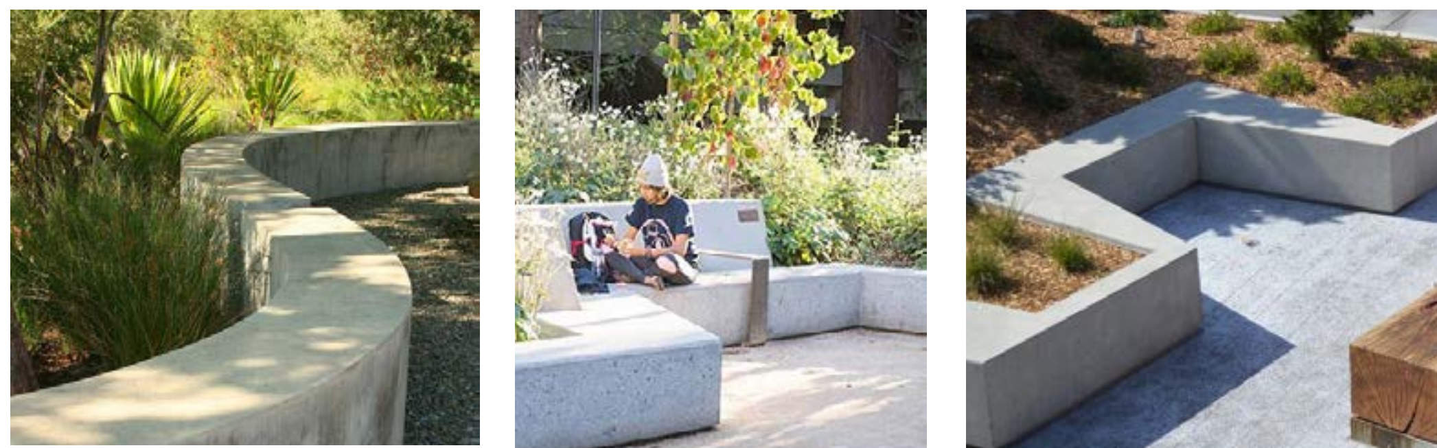
Headhouse planters and Paseo planters will be constructed with concrete at seat height.
