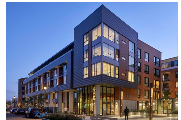
Figure 24: Building Corner at 8th and Fallon Streets
