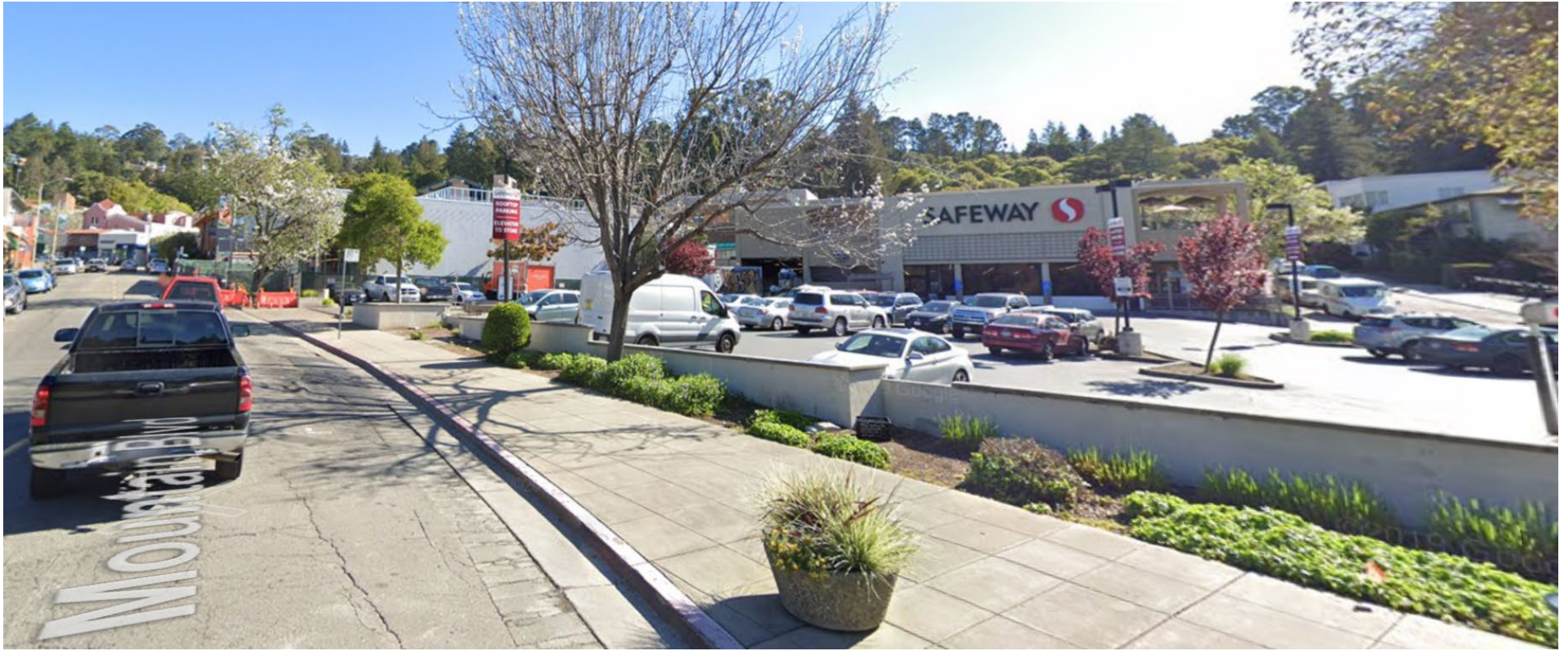
Site of Proposed Site, Looking North on Mountain Boulevard, Side of Building
