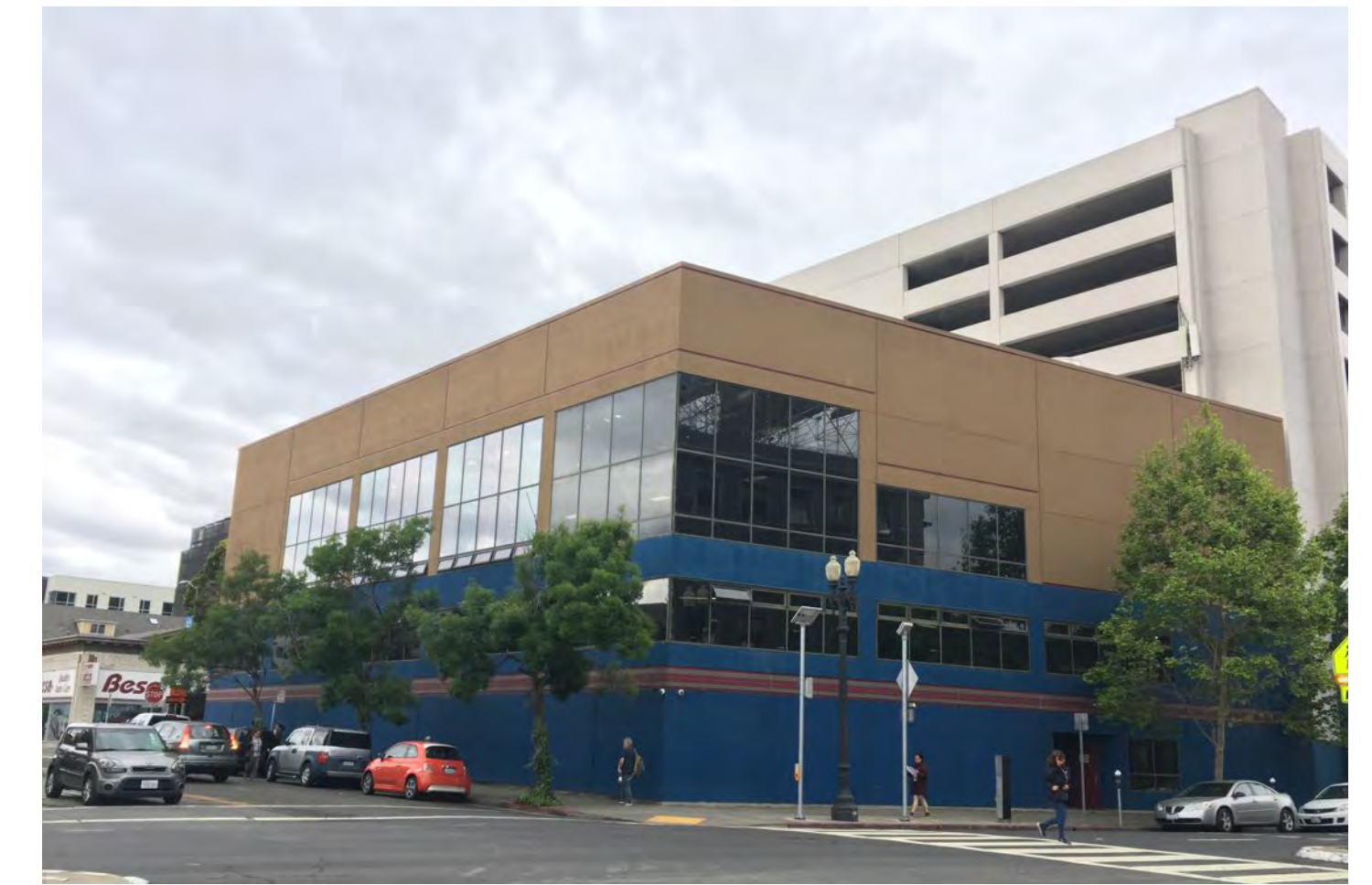
8 24TH ST & WEBSTER: SW CORNER
