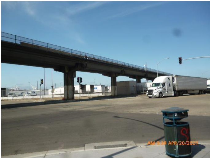
View of a truck on 7 th St. at Wood with USPS trucking facility behind. Many trucks park on 7 th St. and other public streets in the area, whereas the 7 th & Wood site provides off street parking.
