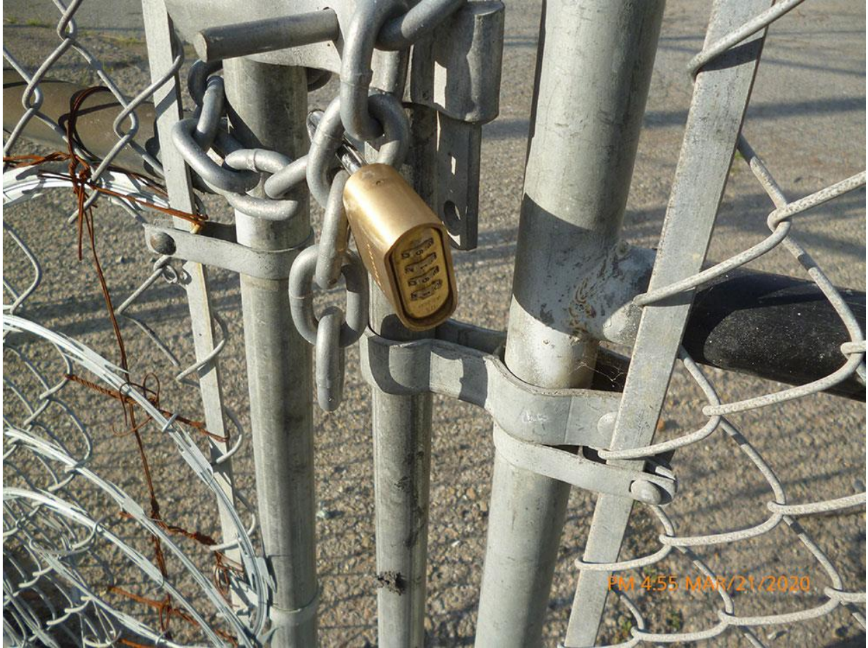
View of the combination lock on 7 th St. for which Owner gave the combination to Gruendl/ Ray's Electric, who changed the combination and left the lock in place to enable trespassing and dumping.
