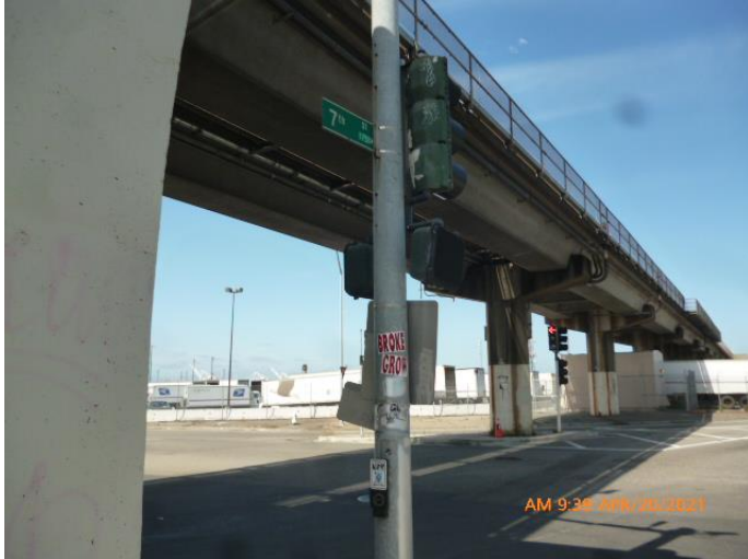
View of the USPS trucking facility looking northwest at 7 th St. & Wood
