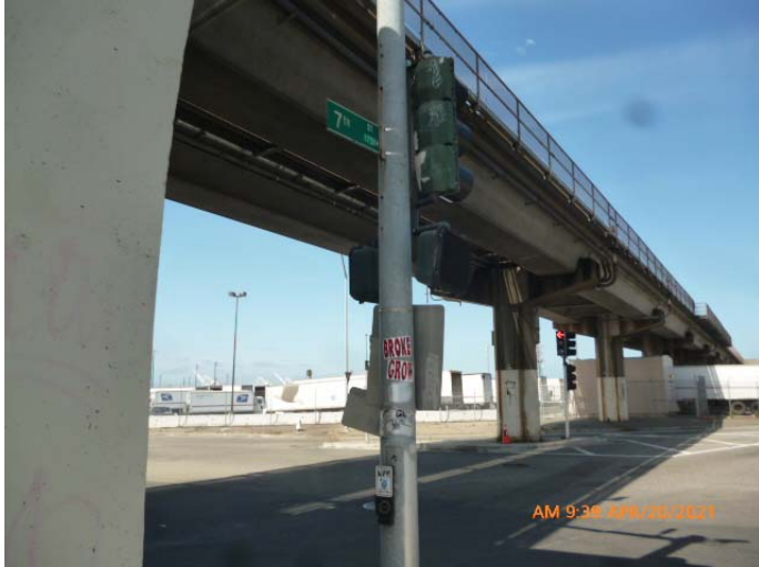
View of the USPS trucking facility looking northwest at 7 th St. & Wood
