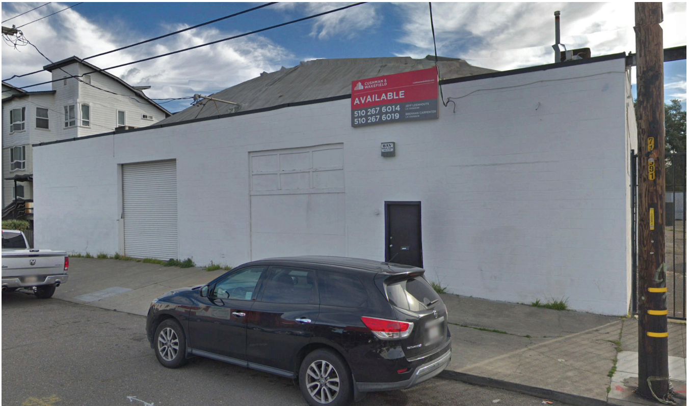
Former Dalzell Industrial Building at 2432 Chestnut Street
