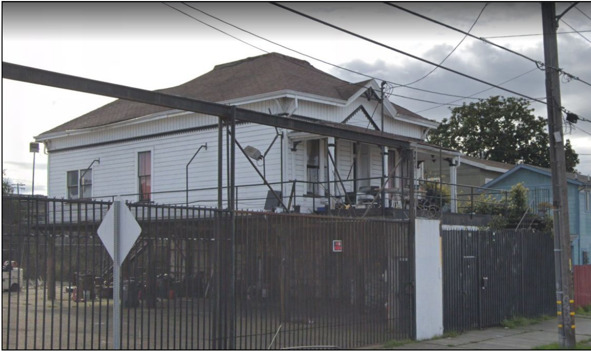
North facade, 2420 Chestnut Street. Source: Google, February 2019.
