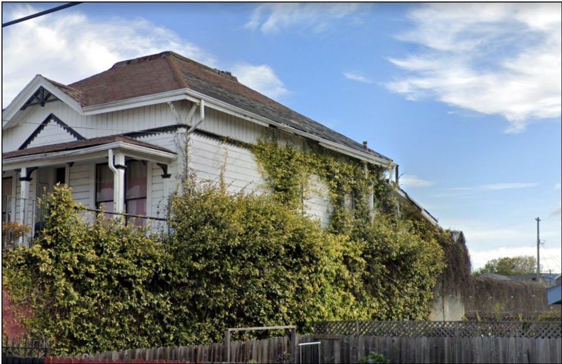
South facade, 2420 Chestnut Street. Source: Google, February 2019.
