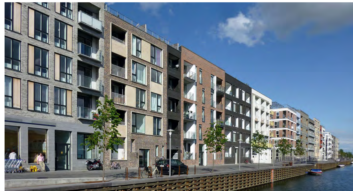
CANAL DISTRICT, SLUSEHOLMEN, DENMARK
