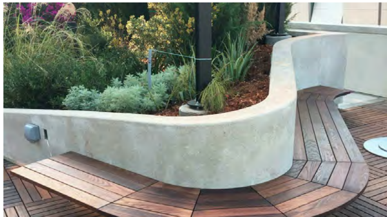
POUR-IN-PLACE CONCRETE WITH SACK FINISH
