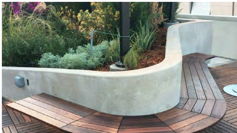
POUR-IN-PLACE CONCRETE WITH SACK FINISH
