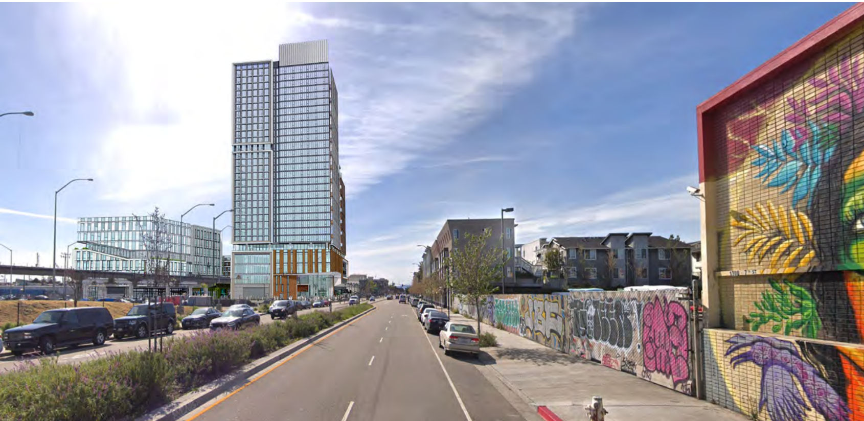
CONTEXT VIEW FROM 7TH STREET LOOKING WEST
