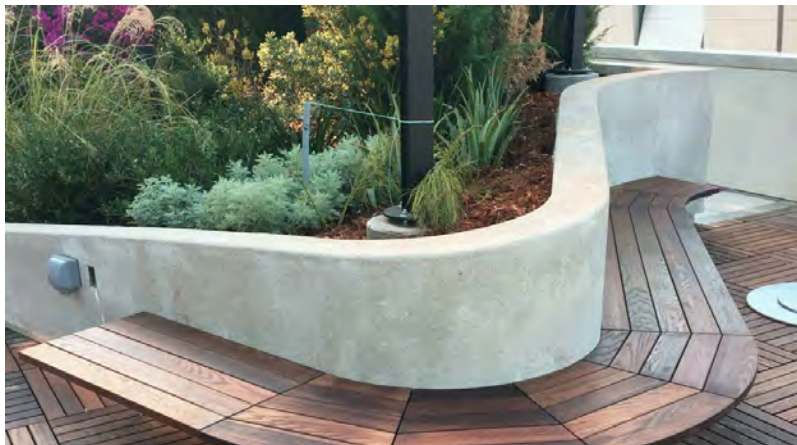
POUR-IN-PLACE CONCRETE WITH SACK FINISH
