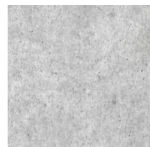
EXPOSED CONCRETE COLUMNS
