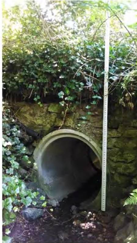
Figure 3: Culvert immediately downstream of the project site.
