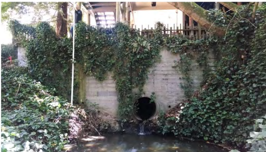
Figure 2: Culvert immediately upstream of the project site.
