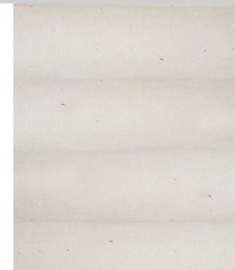
FINISHED ARCHITECTURAL CONCRETE WITH REVEALS
