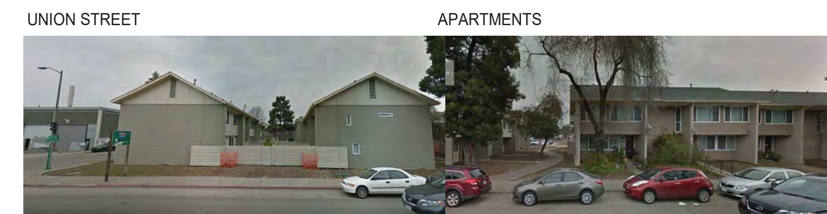
7TH STREET - LOOKING NORTH (CONT.)
