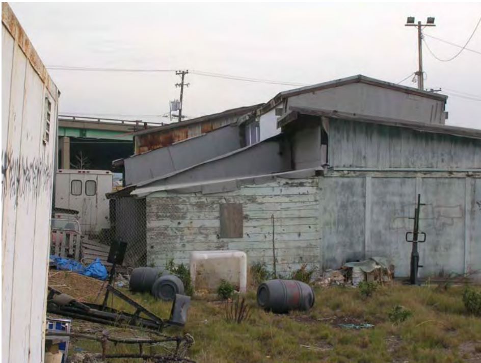
Northwest corner ( Carey & Co. December 2005 )
