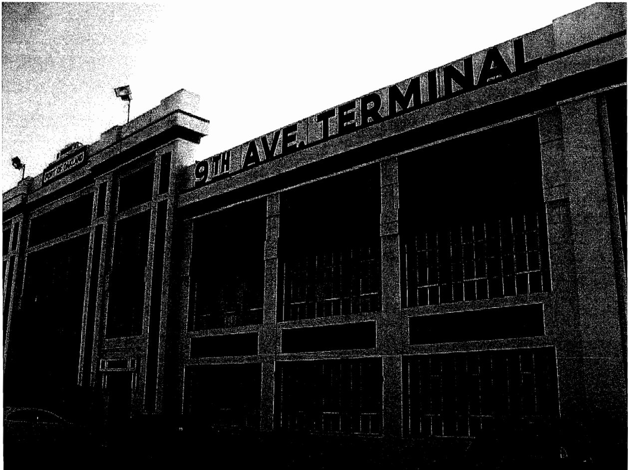
Historic 1929 bulkhead of Ninth Avenue Terminal
