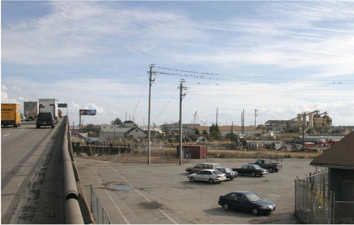
Existing view from Interstate 880 southbound near Oak Street on-ramp looking southeast (VP6)
