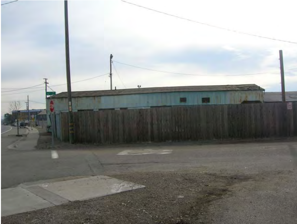
North elevation ( Carey & Co. December 2005 )
