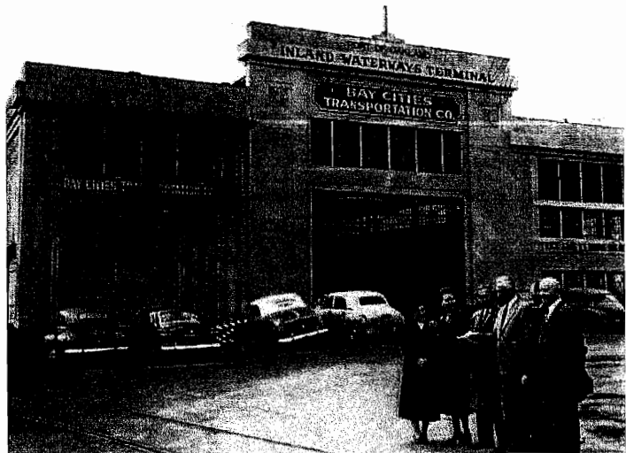
Inland Waterways Terminal - Demolished (Port of Oakland Archives)
