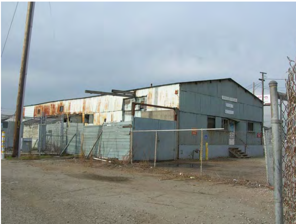
Southeast corner ( Carey & Co. December 2005 )
