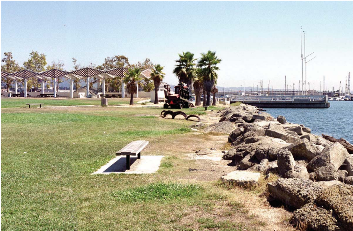
Existing view from Estuary Park shoreline looking east (VP2)
