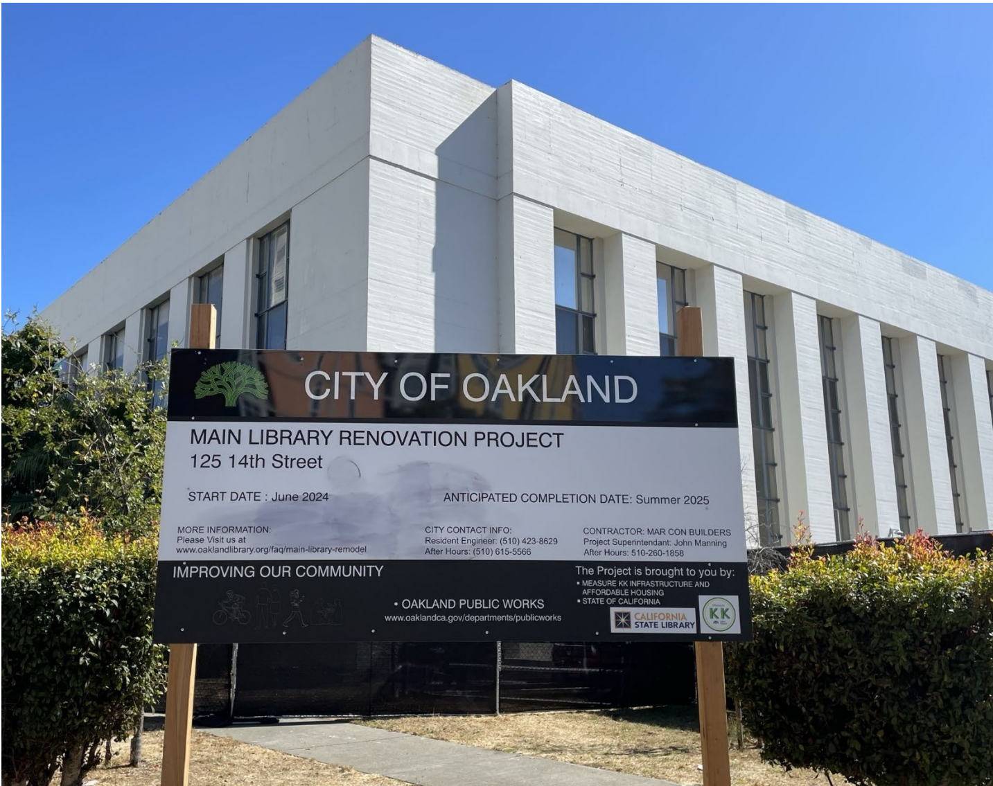
Main Library Renovation
